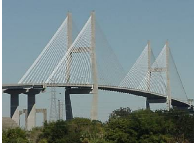
'A' Shape Bridge in Savannah, Georgia
