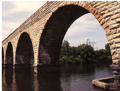
An Arch Bridge in Minnesota
