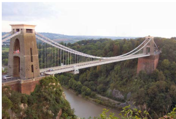
'M' Shape Clifton Suspension Bridge
