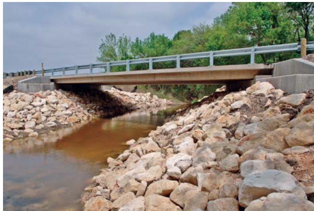
Beam Bridge in Battleground Creek Bridge in Texas
